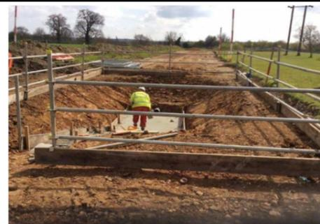
Fig. 2. Typical cable jointing pit from ground level before reinstatement
