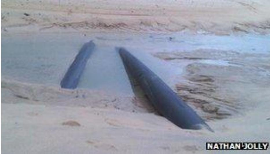
Figure B.6. Wavehub transmission cable exposure on Hayle Beach, Cornwall, November, 2011. From [<http://www.bbc.co.uk/news/uk-england-cornwall-15540281>]
